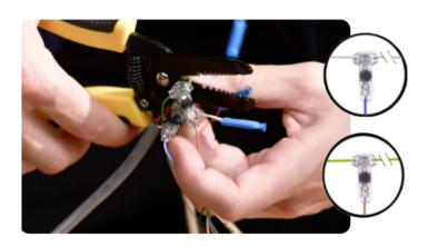
4 Connect the green and white conductors from the panel side harness to the green and white IDCs of the Zerver B wiring harness. Allow for the the end of the conductor to pass through the IDC with a small amount of excess overhang. This will insure that the splice makes adequate contact between conductors.
